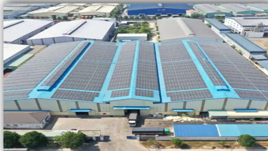
My Phuoc: 1.200 KWp
